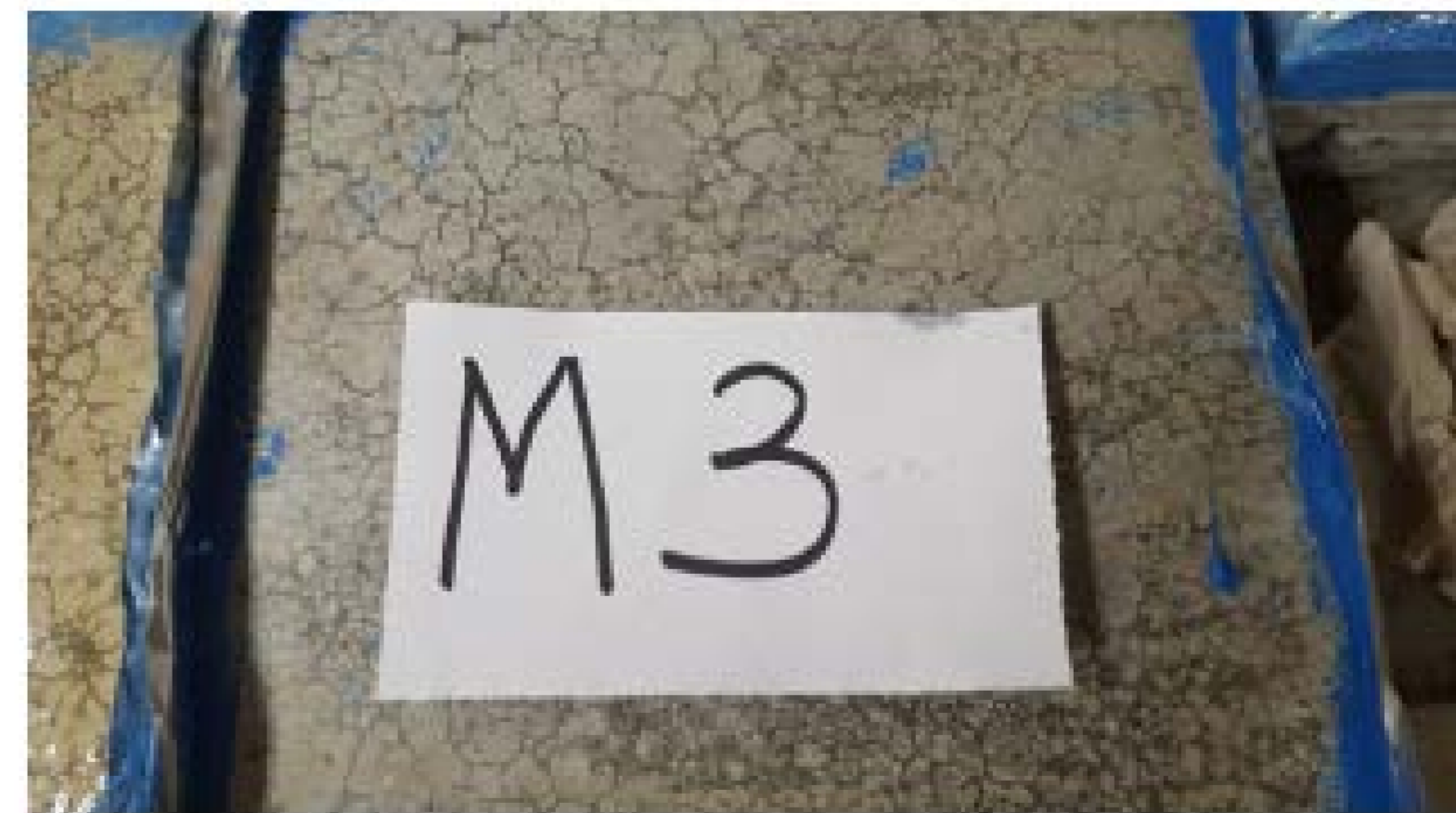
Figure 10: Thain road paving Lewiston mixture after deicing scaling test
