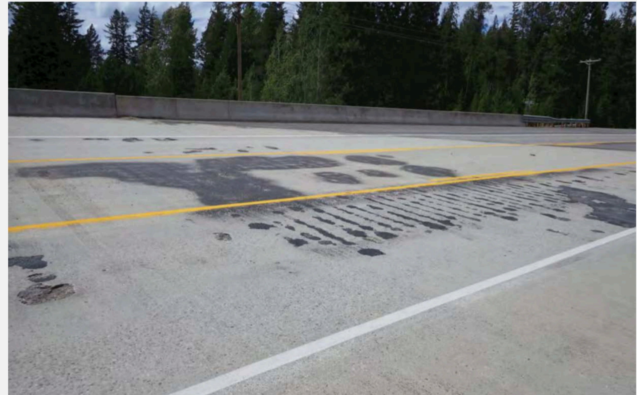
Large area of patched spalls, spalls with rebar exposed and delamination at mid-span of deck.
