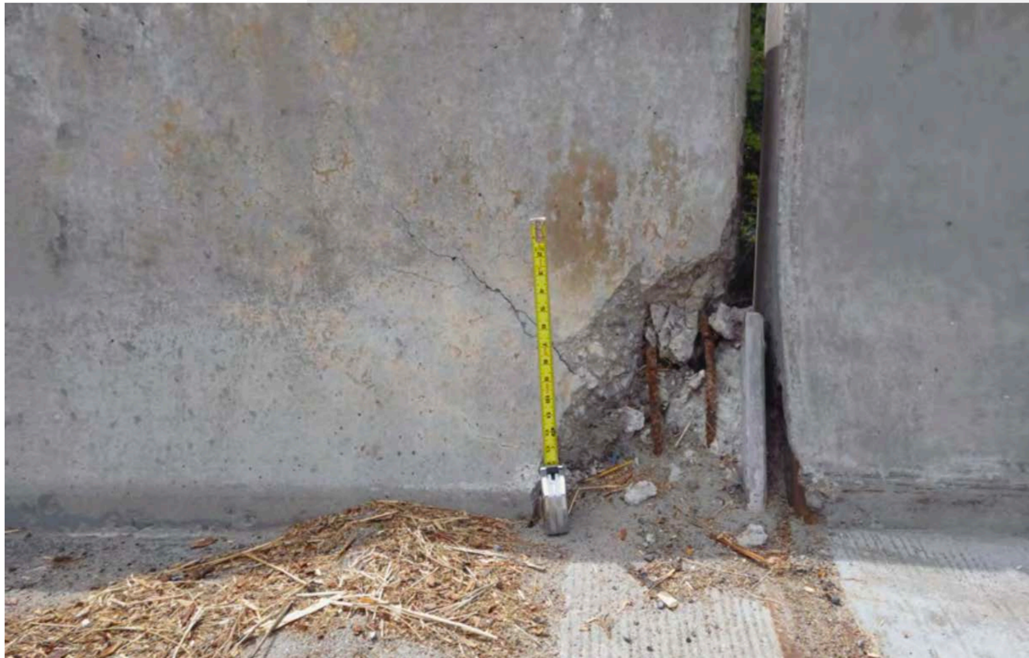
Spall in approach rail at SW. (ITD 2012)
