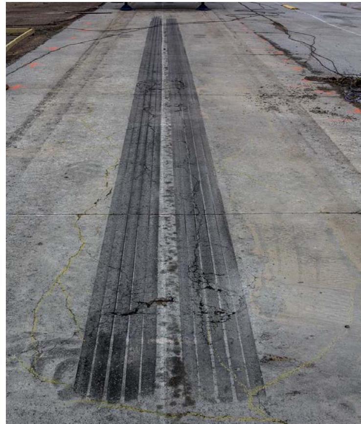
Pavement Condition at the end of testing
