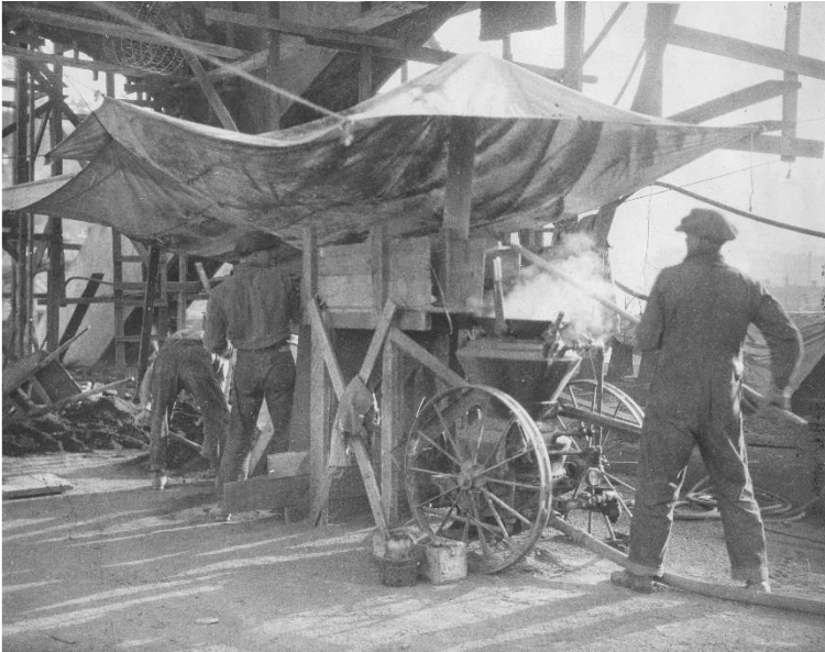
Dual chamber Shotcrete gun 1922
