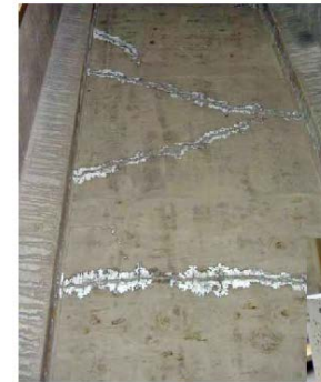
Full-Depth Shrinkage Cracking on Prestressed Girder Bridge
