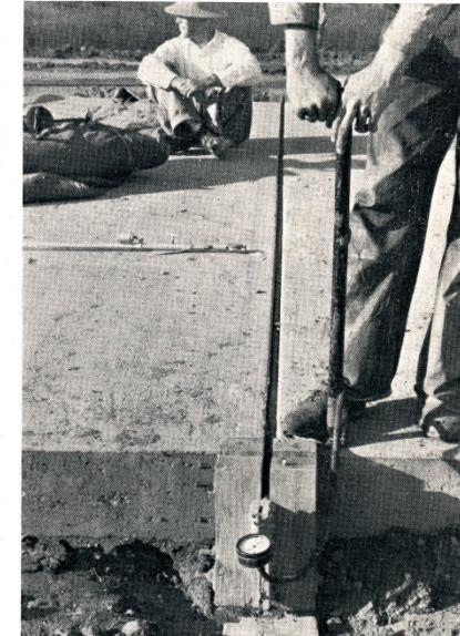
*View of transverse joint showing the hose in the joint, the clamps and pressure gauge, and pressure being applied with an ordinary tire pump. Pressures up to 150 pounds per square inch were readily obtained.*
