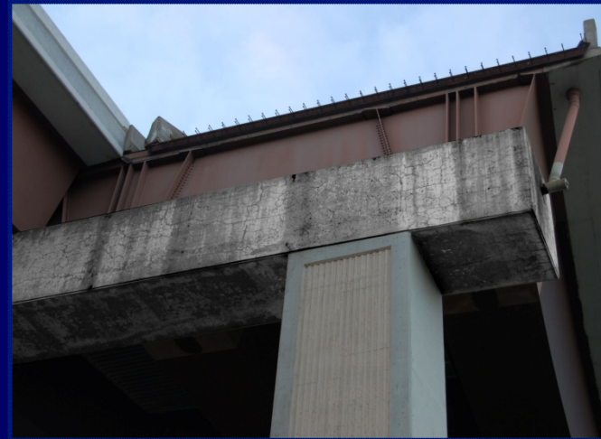
US 59 & I-10 Interchange
