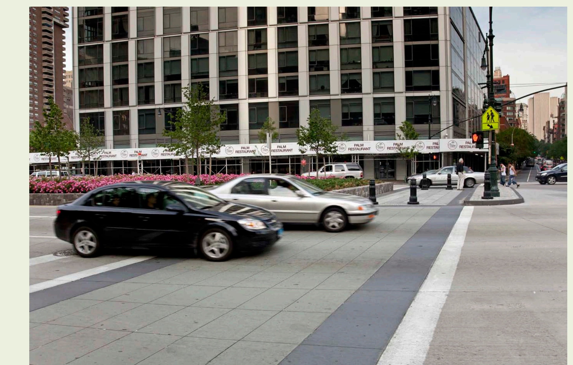
PCC Pavement Rebuilds Lower Manhattan
