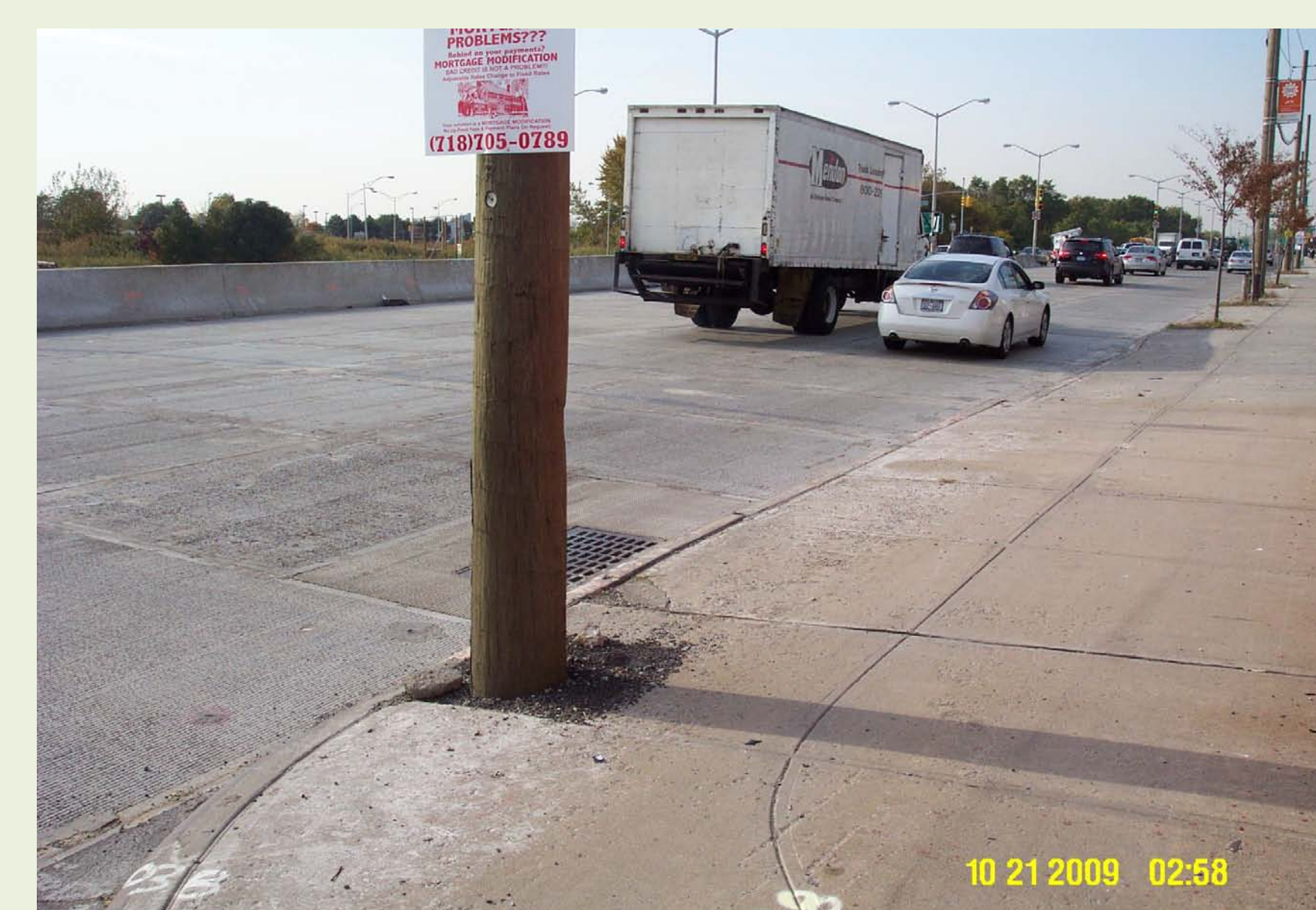
Precast PCC Pavement
