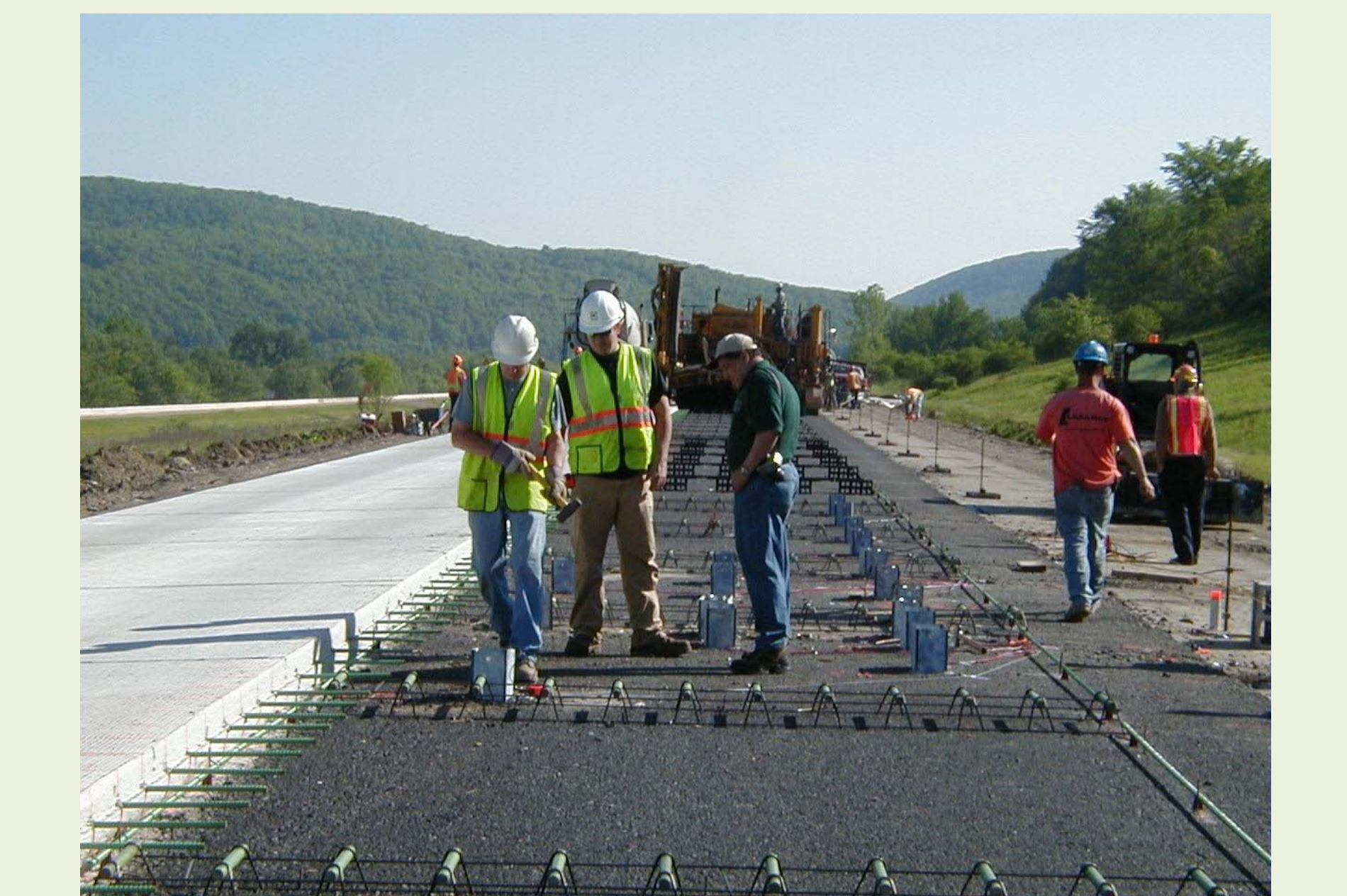
Unbonded PCC Overlay Test Section Atop Rubblized, Cracked and Seated, and Non-Fractured PCC Pavement
