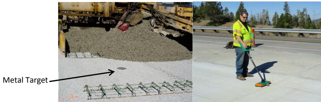
Iowa DOT has realized the benefit of using the MIT Scan T2 and has been using it as part of their specifications since 2010. Several FHWA field trials have shown that the MIT Scan T2 works well over a wide range of concrete pavement thicknesses and base conditions.
