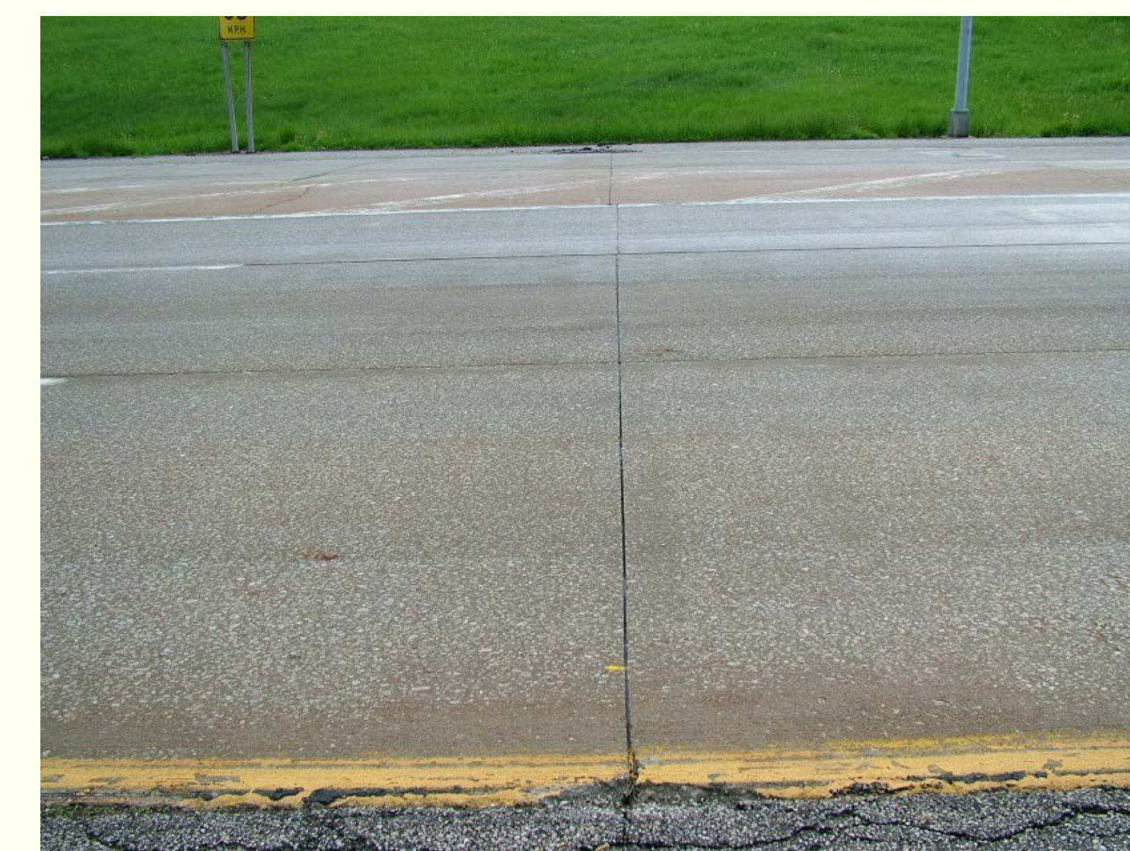
Figure 2. Photo of surface condition of pavement with plastic-coated dowels (State Route 59)
