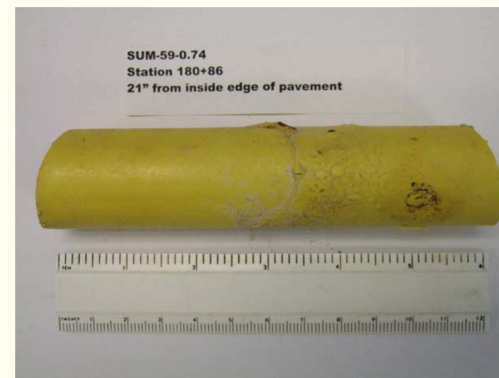
Figure 1. Photo of plastic-coating of dowel on State Route 59 after 33 years of service
