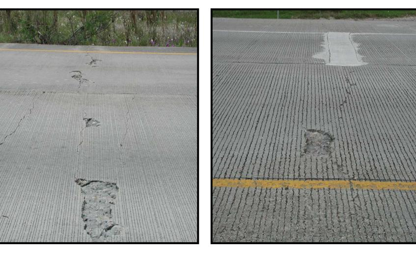
Figure 1: Typical Shallow Spalling in CRCP
