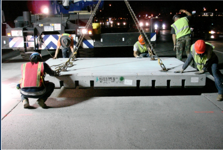
Center Slab in Hole (Single Slab Holes)
