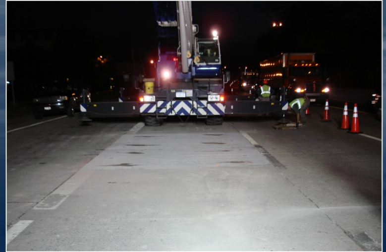
Crane Occupies New Slab
