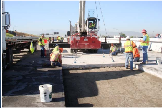
Crane Occupies New Slabs
