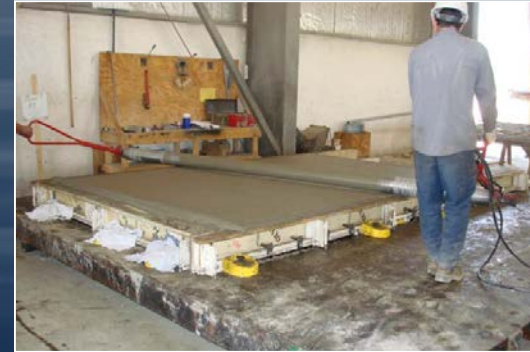
Roller Screed - Accurate Top Surface
