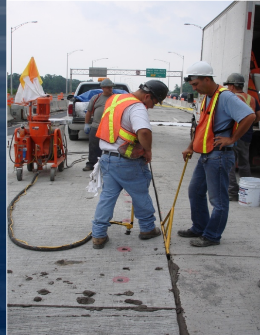
Contractor-Designed Joint Dam
