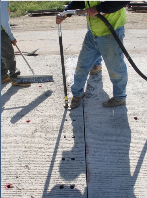
Fill Dowel Slots and Joints First
