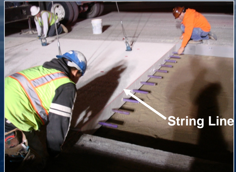
Set Slab to String
