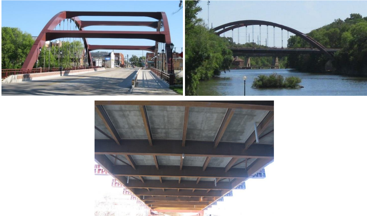
Figure 16. US 65 Bridge over the Iowa River in Iowa Falls: view toward the north near downtown (top left), profile view over the Iowa River looking east (top right), and lower level of the superstructure of the bridge including floor beams, stringers, and deck (bottom)
