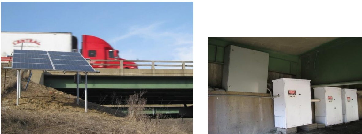
Figure 5. Solar panels providing power to bridge sensors (left) and battery storage cabinets under the bridge (right)
