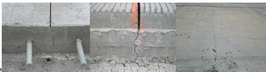
Figure 8-23. Close-up of different degrees of raveling caused by joint sawing (ACPA)
