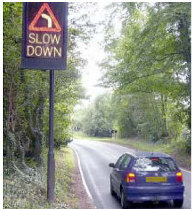
Figure 3: DSFS on curve in the UK (© TRL (Transport Research Laboratory) 2002, from Winnett and Wheeler 2002)
