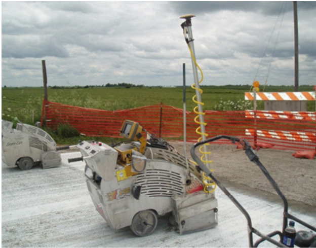
Saw equipped with a GPS unit in Poweshiek County
