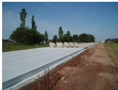
Finished pavement in Osceola County
