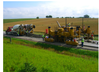
Two-lane stringless paving in Poweshiek County
