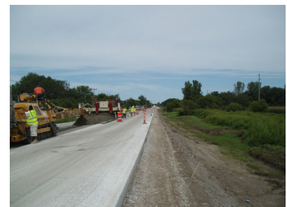
Single-lane paving with stringline in Johnson County
