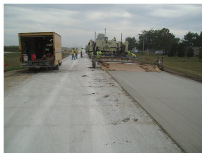
Single-lane stringless paving in Worth County
