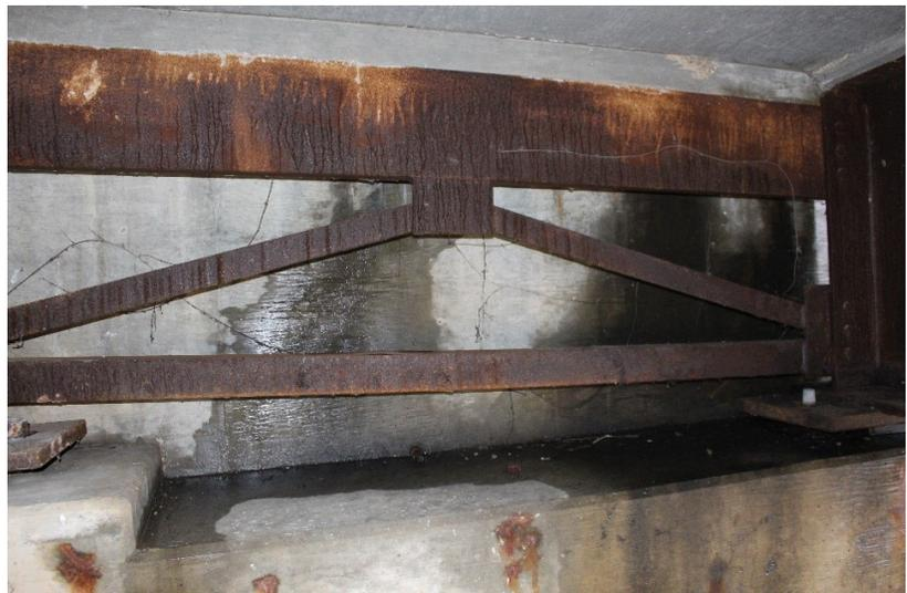
Corrosion damage caused by a leaking joint
