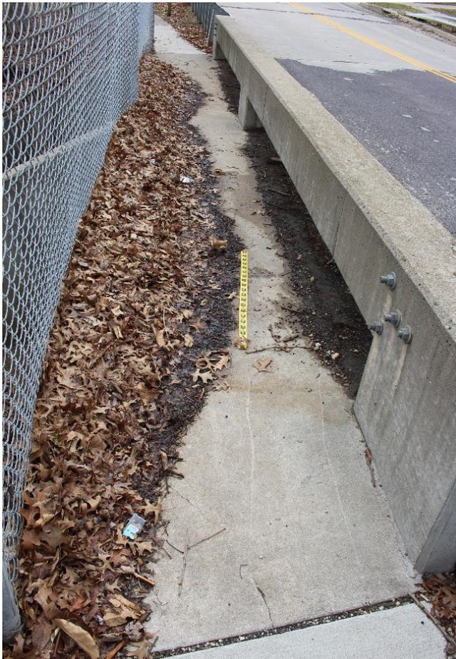
*Debris accumulation that can cause corrosion and spalling*
