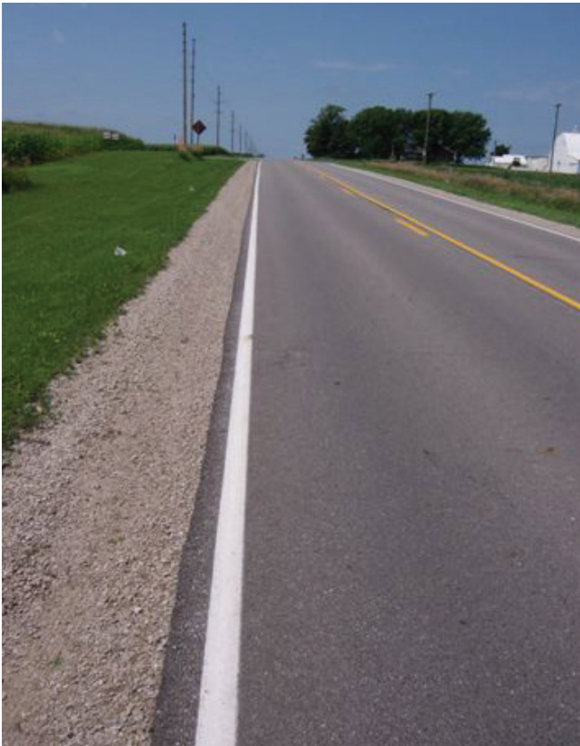
Responses to the pavement-marking survey showed that most of the paved secondary roadways in Iowa have both centerline and edgeline pavement markings as opposed to centerline/no passing zone only (Image: Bob Sperry, retired from Iowa LTAP)
