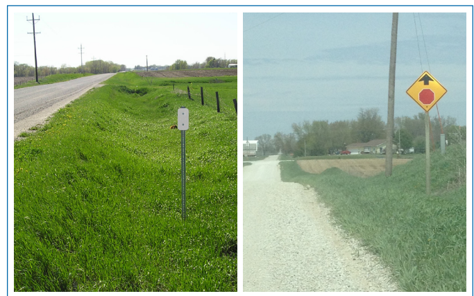
Sample Mitigation: New, highly-reflective delineators and signs installed in Dallas and Story counties
