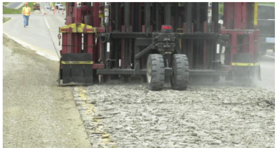
Rubblization using a multiple-head breaker
