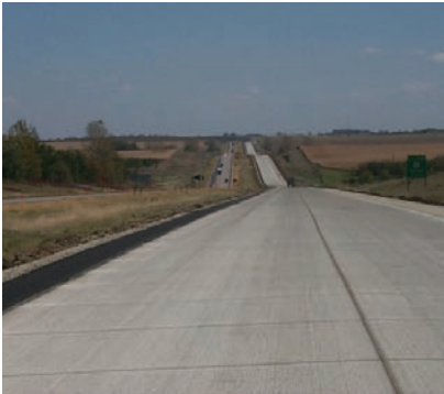
Concrete overlays
