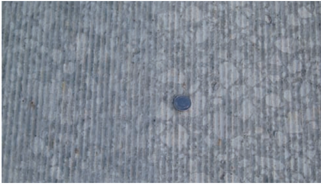
Diamond ground pavement
