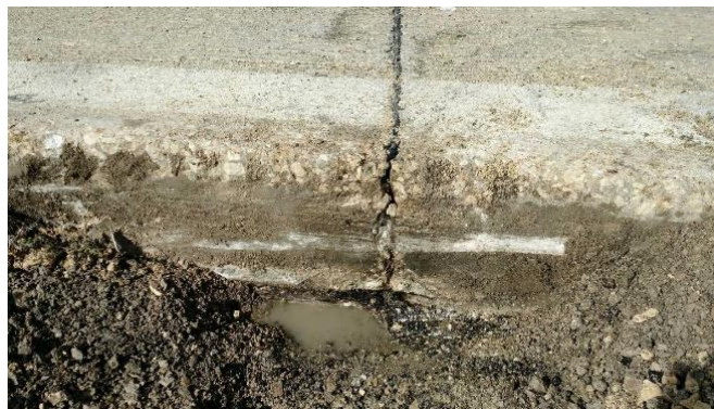
Figure 78. Crack deployment in joint adjacent to blowup
