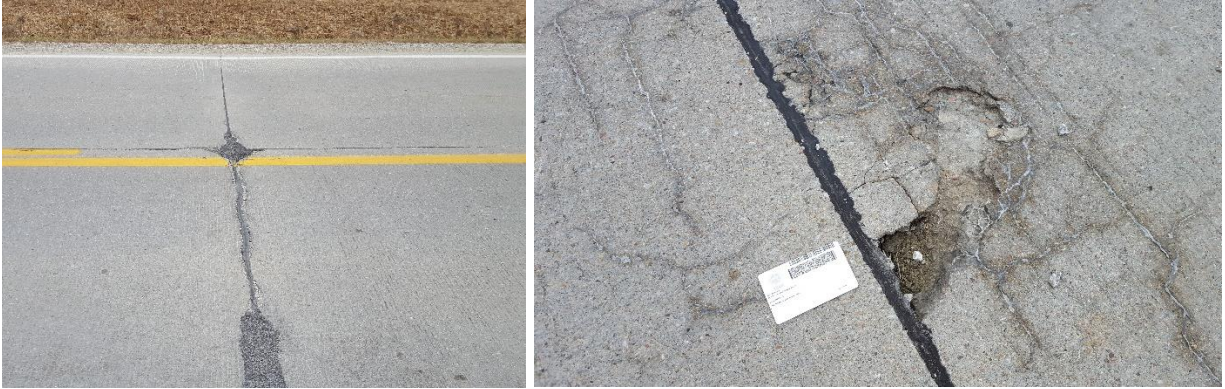
Figure A.44. Apparent material-related distresses at joints on Pottawattamie County L-34, November 2016
