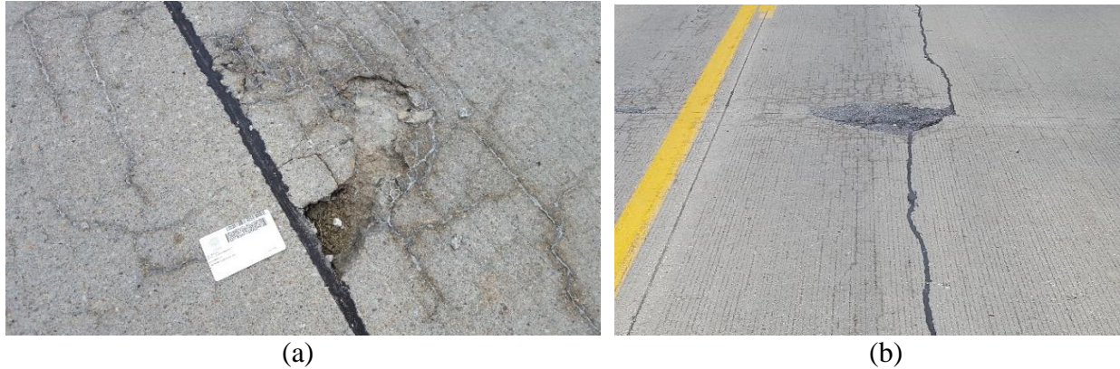
Figure 75. Material durability-related distresses on (a) Pottawattamie County L-34 and (b) Pottawattamie County L-66 (November 2016)
