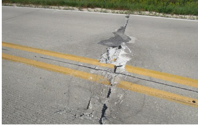
Figure 77. Joint deterioration on North 10th Street in Linn County (September 2016)
