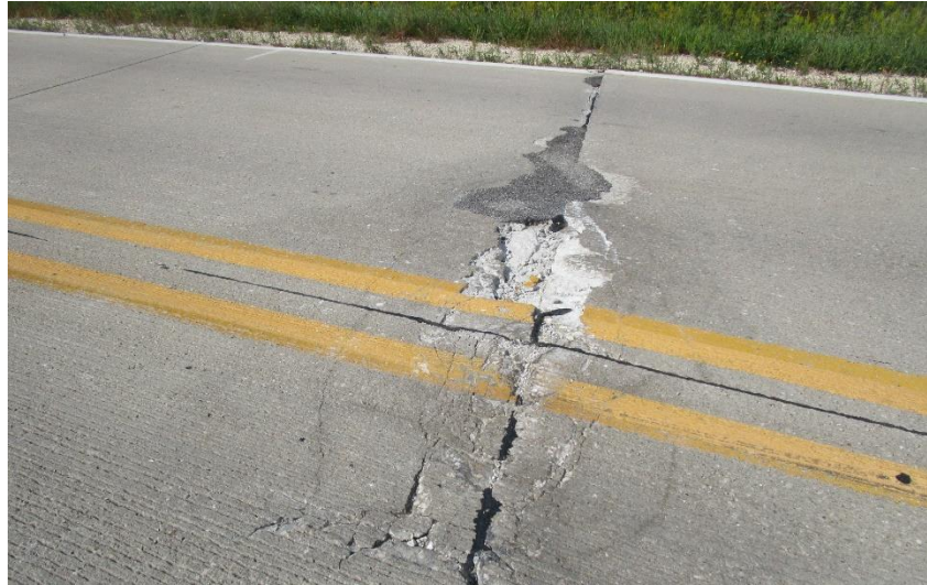
Figure A.36. Joint deterioration on Linn County North 10th Street, September 2016
