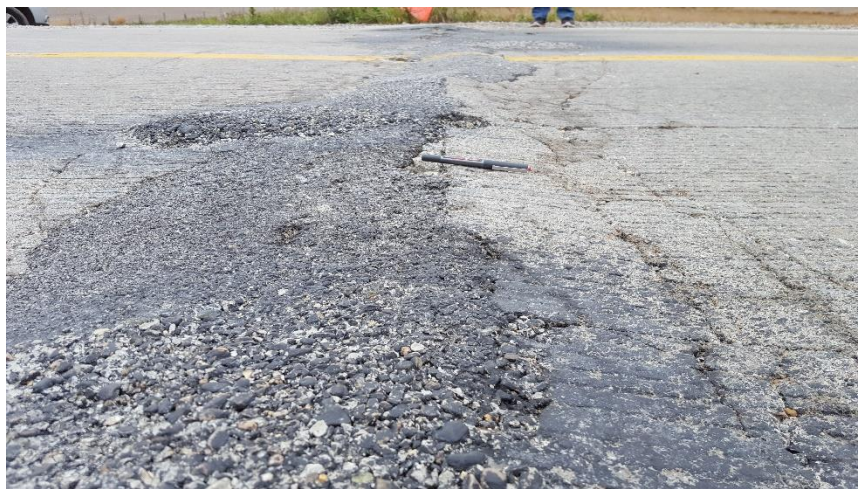
Figure A.49. Apparent blow-up on Pottawattamie County L-66, November 2016
