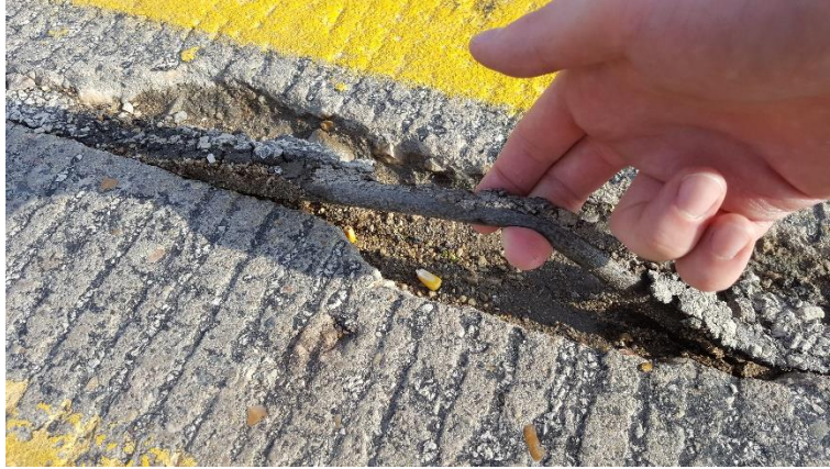
Figure A.23. Deterioration around and underneath the backer rod on Dallas County F-31 west of Minburn, November 2016
