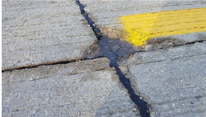
Figure A.18. Water at spalled joint and adjacent joint shadowing on Dallas County F-31 west of Granger, November 2016
