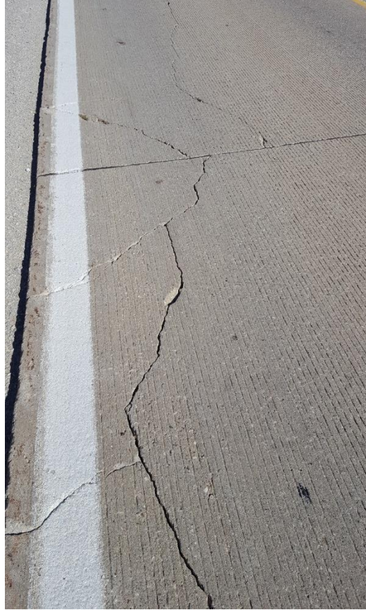
Figure A.11. Longitudinal and corner cracking at slab edge in southbound lane of Buchanan County W-40, September 2016
