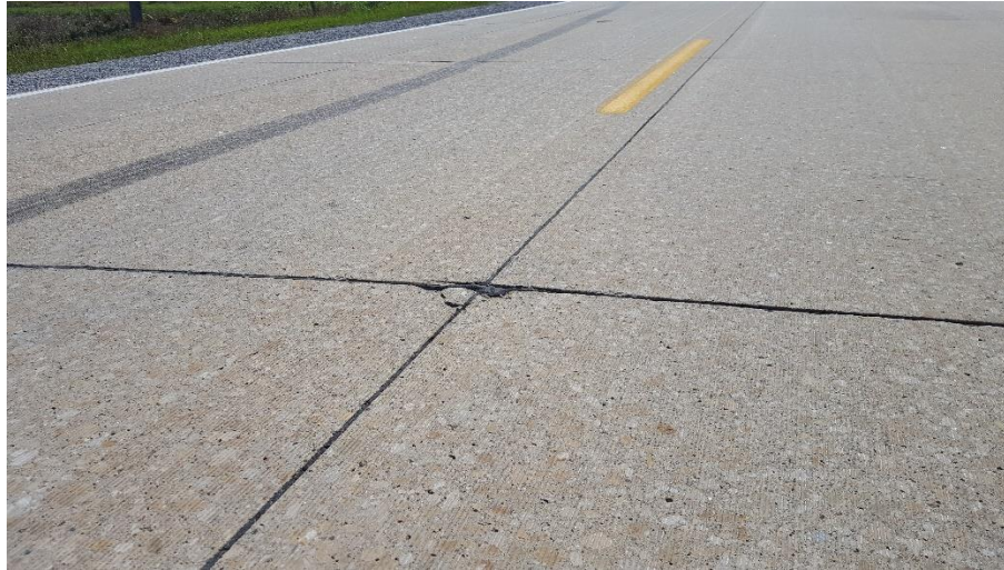
Figure A.5. Surface post diamond grinding on Buchanan County V-62, September 2016
