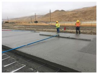
Figure 3. Typical Hand Finishing Procedures
