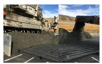
Figure 2. Concrete Dumped Directly in Front of the Paver Using Belt Placer
