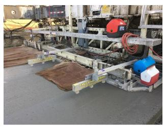
Figure 1. RTP Installed Directly at the Rear of the Paver
