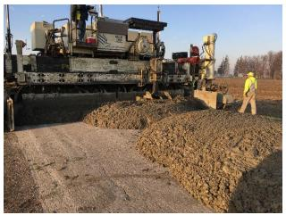
Figure 3. Concrete Dumped Directly in Front of the Paver
