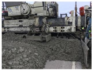
*Figure 6. Relatively High Level of Concrete at the Front of the Paver*
