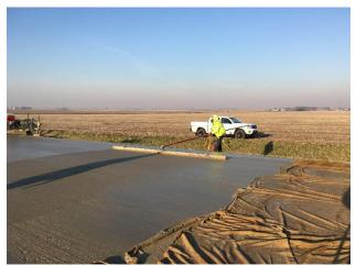
Figure 2. Typical Finishing With a Straightedge
