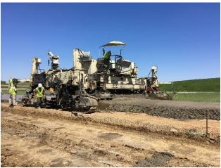
Figure 4. Concrete Spread Ahead of the Paver
