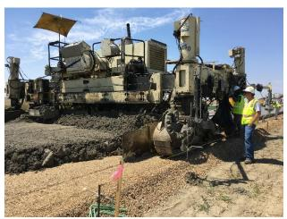
Figure 5. Stable and Trimmed Paver Track Line
