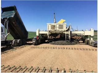
Figure 3. Belt Placer/Spreader Ahead of the Paver
