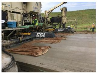
Figure 1. GSI Installed Directly at the Rear of the Paver
