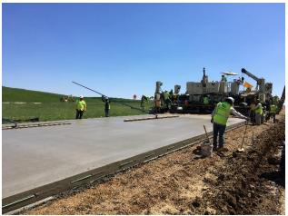
*Figure 2. Typical Hand Finishing With a Straightedge and Channel Mop*
