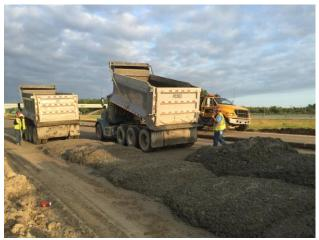
Figure 2. Concrete Deposited on Grade Ahead of the Paver
