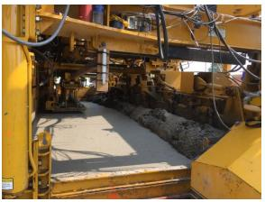
Figure 4. DBI Section of the Paver Showing the Oscillating Finisher
