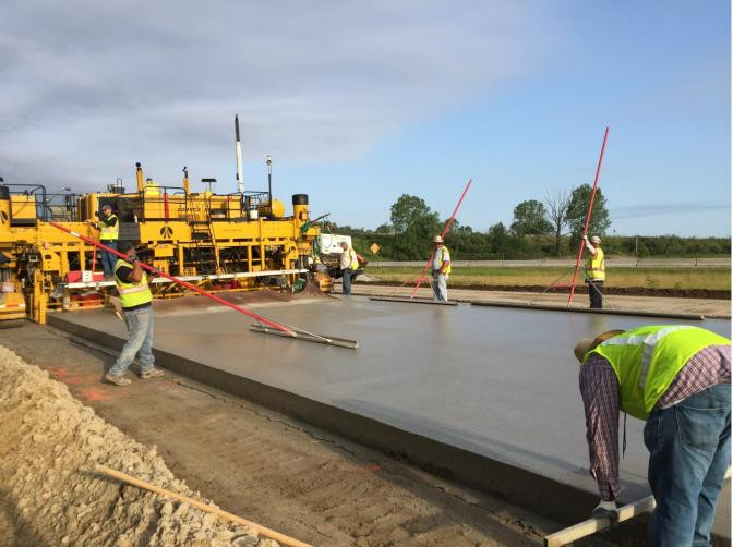
Figure 7. Stable Edges and No Surface Voids Directly Behind the Paver
