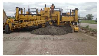
*Figure 2. Concrete Deposited on Dowel Baskets Ahead of the Paver*
