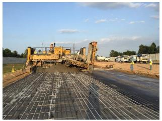
*Figure 2. Concrete Spreading by Gomaco 2600 Ahead of the Slipform Paver*
