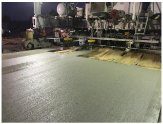
Figure 1. Gomaco GSI Mounted to G-Z S-850 Paver With a Float Pan
