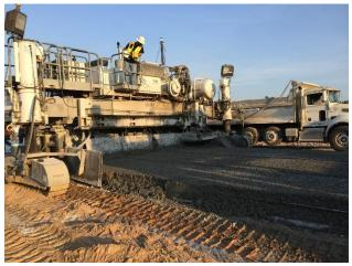
*Figure 3. Concrete Deposited on Reinforcing Steel Ahead of the Paver*
