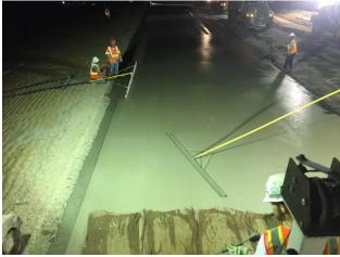
Figure 4. Typical Hand Finishing Behind the Paver
