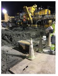
Figure 4. Paving at a Drainage Structure
