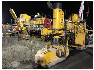
*Figure 2. Concrete Dumped Directly in Front of the Paver*
