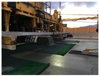
*Figure 1. GSI Installed Directly at the Rear of the Paver*
