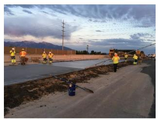
*Figure 3. Typical Finishing Hand Finishing Behind the Paver*
