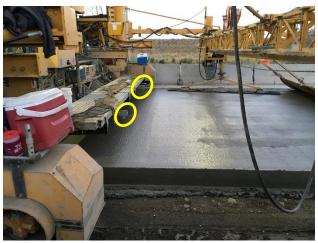
*Figure 1. RTP (yellow ovals) Installed Behind the Dowel-Bar-Inserter (with OCB).*
