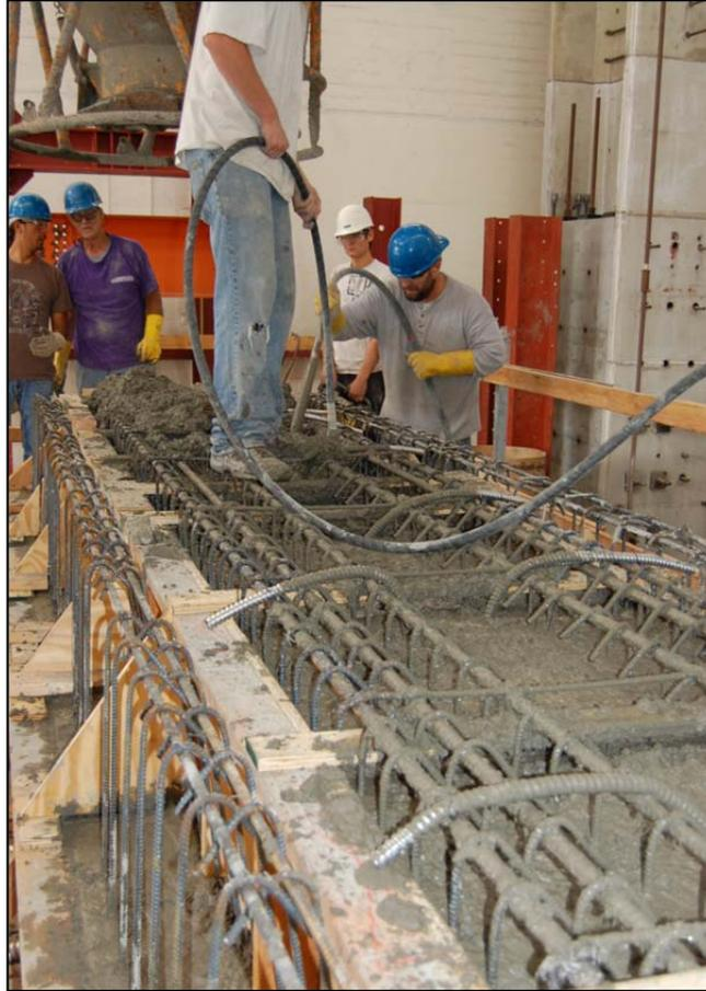
Figure 5.8: Casting of the Bent Cap
