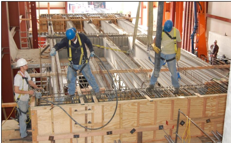
Figure 5.6: Casting of the North Abutment
