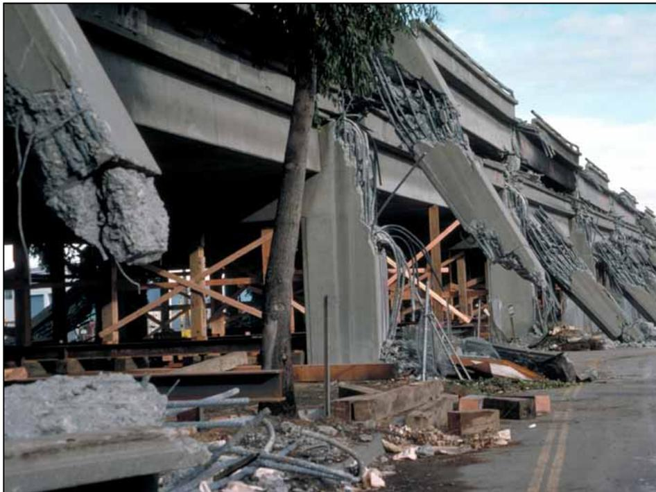
Figure 1.2: Example of 1989 Loma Prieta Earthquake Damage (*Courtesy of UCSD*)
