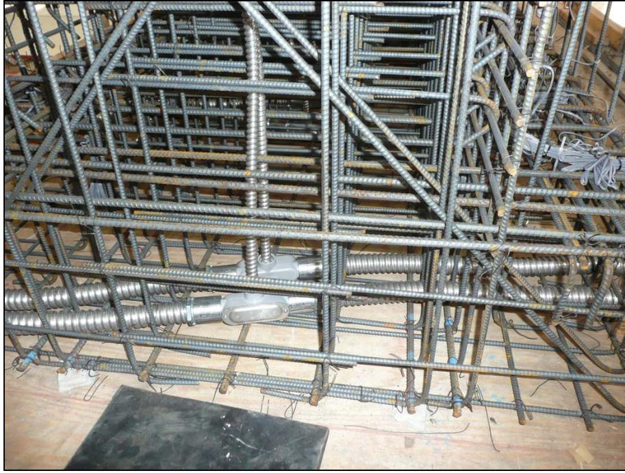
Figure 5.9: Routing of Bent Cap Ducts
