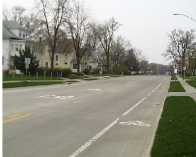
Figure 6. Three-Lane Cross Section with Bike Lanes.
