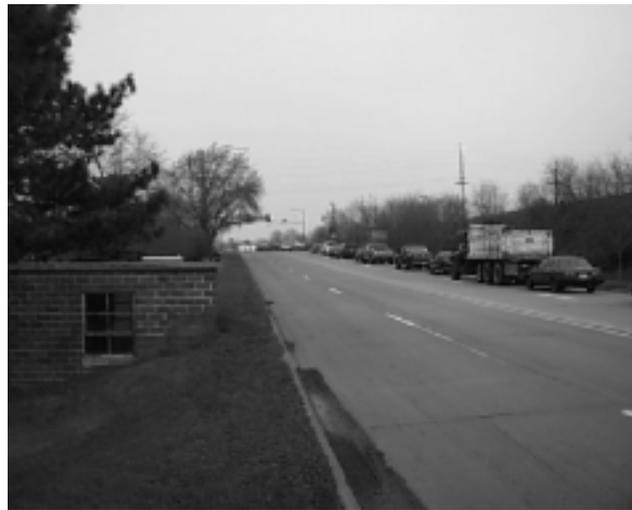
**Figure 4 Four-lane Undivided Roadway/Intersection Operating as a “Defacto” Three-Lane Cross Section**
