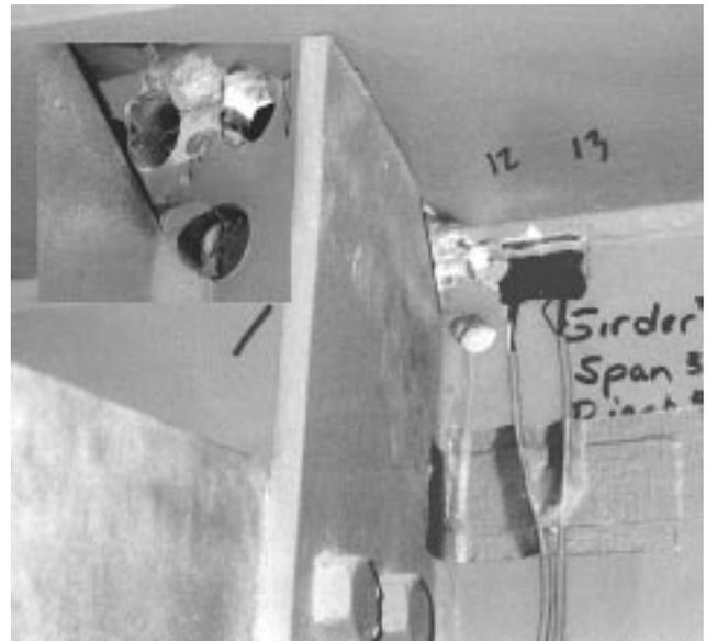
FIGURE 4 Cracks and drilled holes at Location H.
