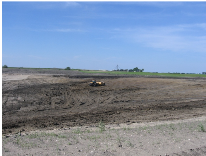
Figure 5. New construction site for U.S. 20 in Calhoun County
