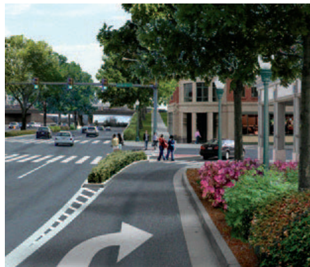
Figure 1. Channelized right turn lane (Urban Advantage, CD+A, and H.B. Rue for the Thomas Jefferson Planning District Commission, Albermarle County, and Virginia DOT, from Grant et al. 2012)
