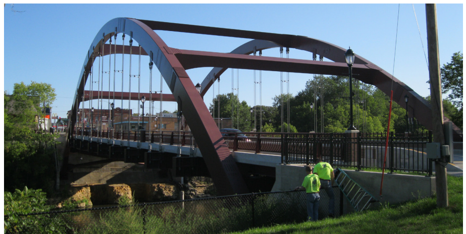
Iowa Falls Arch Bridge, which the researchers instrumented during and after construction for installation, implementation, and operation of the pilot continuous monitoring system
