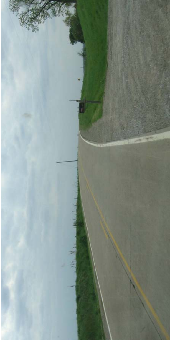
Figure C.3. Combination horizontal and vertical curvature
