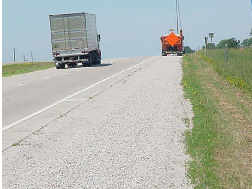
Figure 5. Stationary Iowa DOT Truck on the Shoulder at a Crest Vertical Curve
