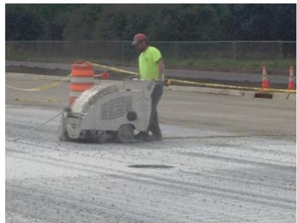
*Typical early entry saw-cutting process*
