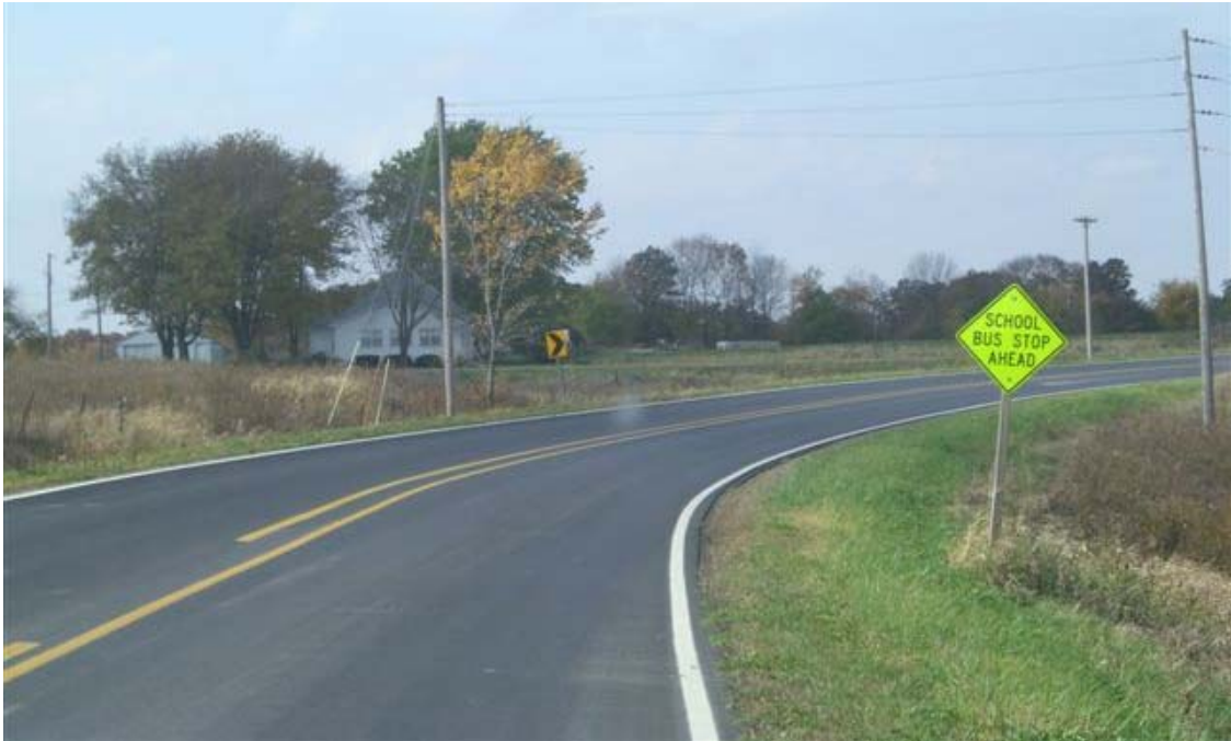
Figure A.1. School bus warning sign and chevron along horizontal curve at Palm Boulevard intersection
