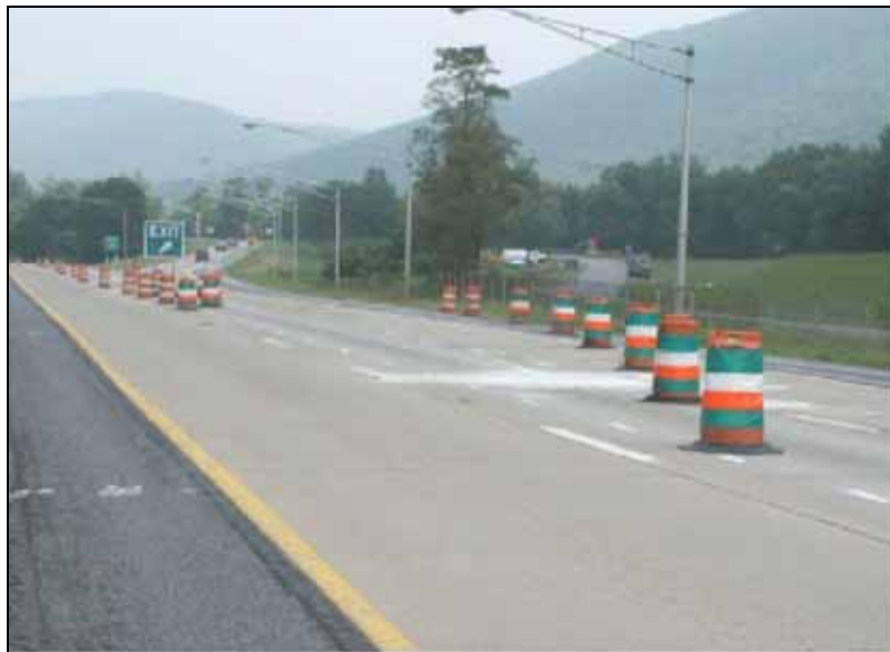
Figure 4. Alternate-colored drums at exit taper (PennDOT)
