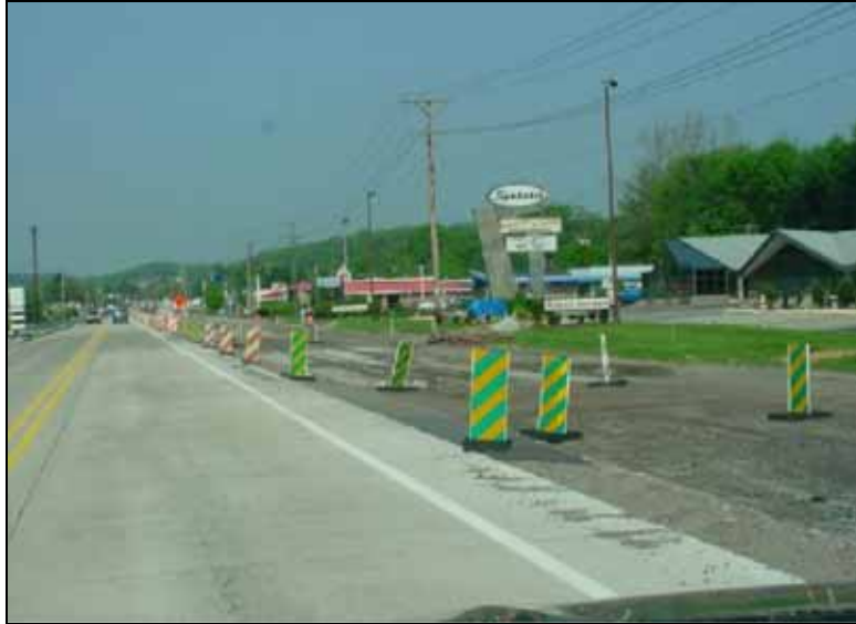
Figure 3. Alternate-colored vertical panels at entrance taper (PennDOT)
