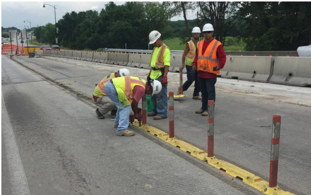
**Figure 1. Temporary bollards being detached by workers**
