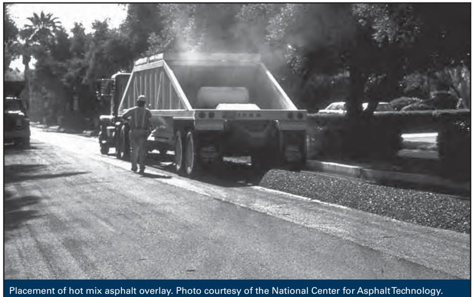
Placement of hot mix asphalt overlay. Photo courtesy of the National Center for Asphalt Technology.
