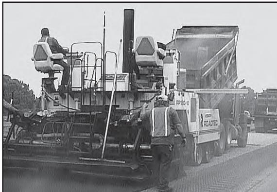
A hot mix asphalt laydown machine with constant flow of materials helps ensure paving uniformity. Photo courtesy of the National Center for Asphalt Technology.
