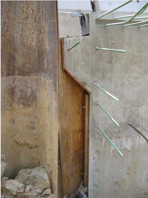
*Inclined paving notch observed during construction of a new bridge*
