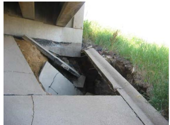
*Failure of concrete slope protection due to erosion*
