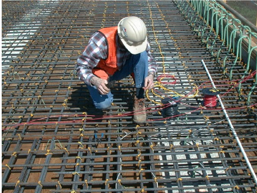
Figure 3.10. Extending lead wires for data measurement
