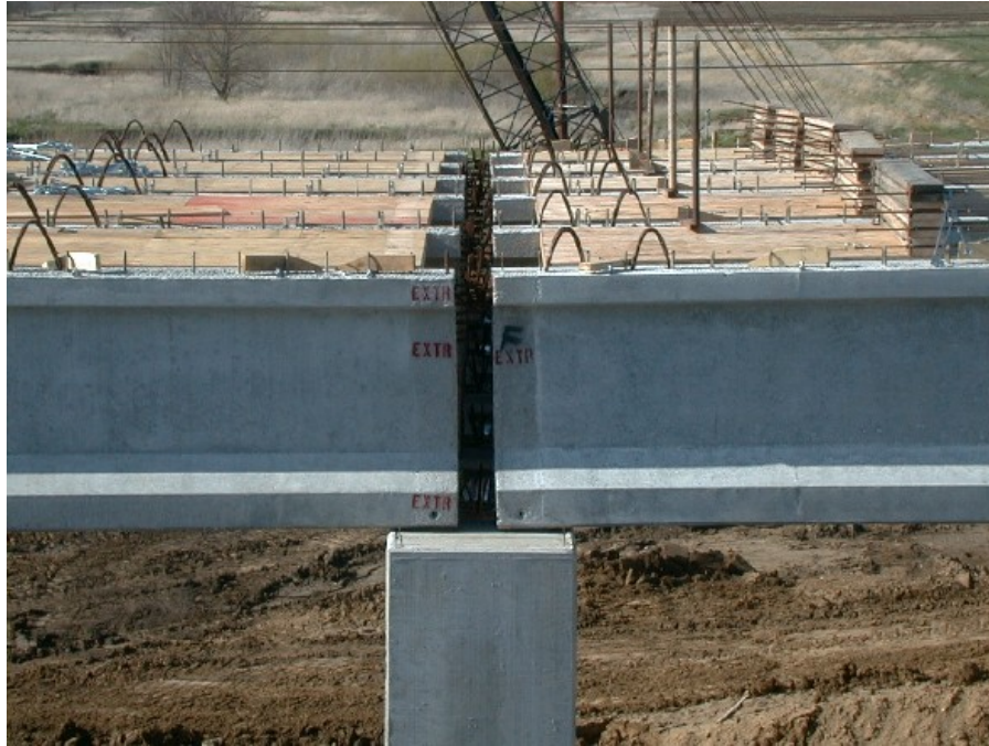
(c) Typical beam connection at pier Figure 3.2. Typical prestressed I-beams
