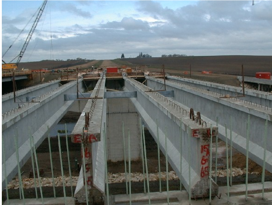
(a) Typical beam layout
