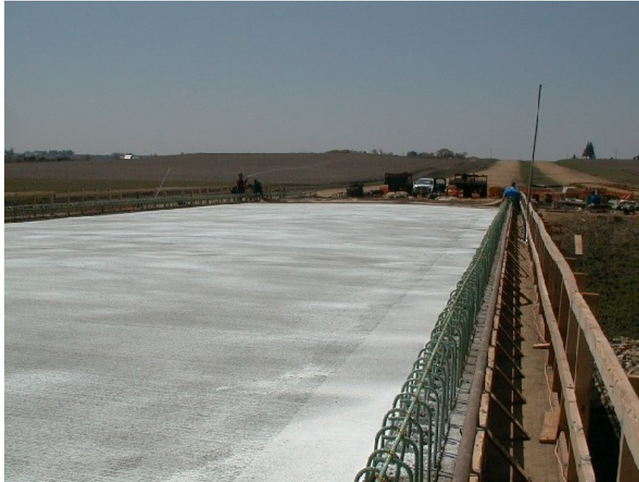
Figure 3.5. Bridge deck concrete placement completed
