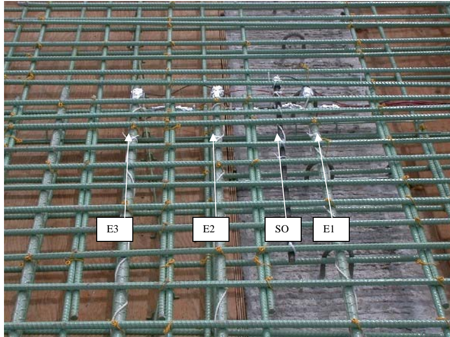
(a) “SO” MMFX bar and epoxy bars E1–E3 (looking east)
