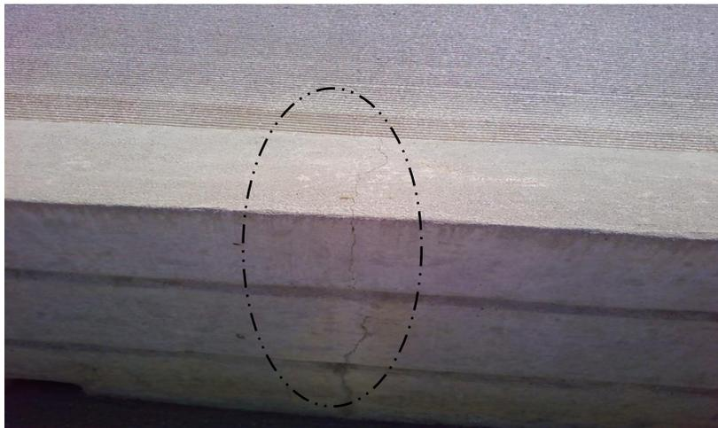
**Figure 4.5. Guardrail transverse cracking**
