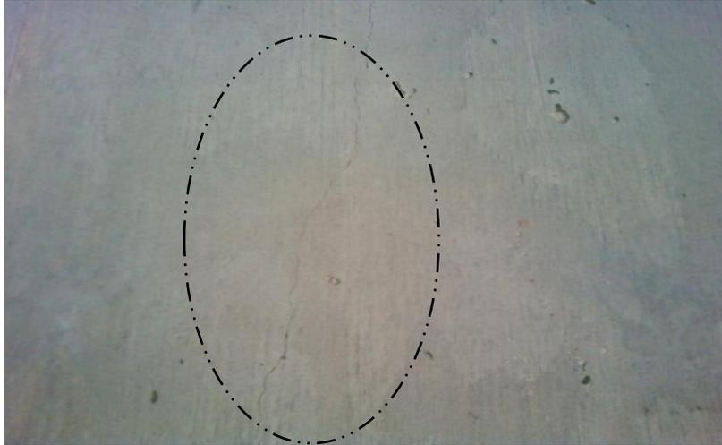
**Figure 4.1. North abutment hairline crack**
