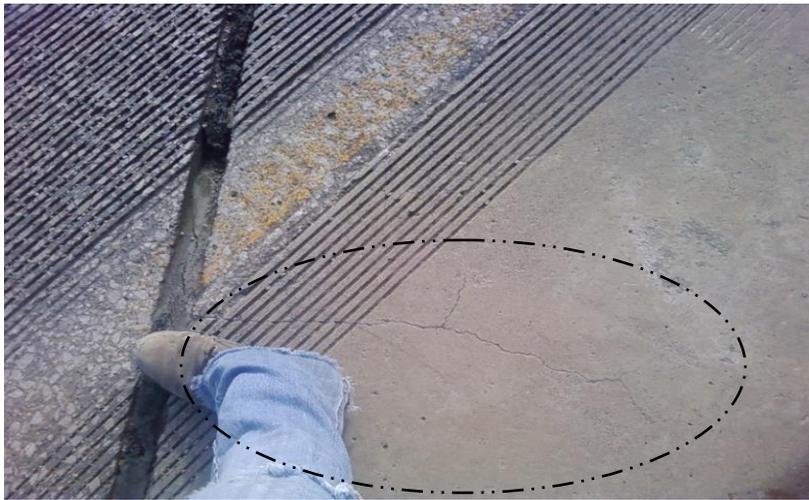
**Figure 4.3. Off-ramp slab cracking**
