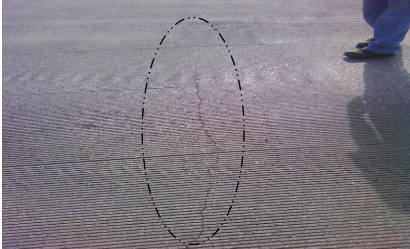
**Figure 4.4. Deck transverse cracking**
