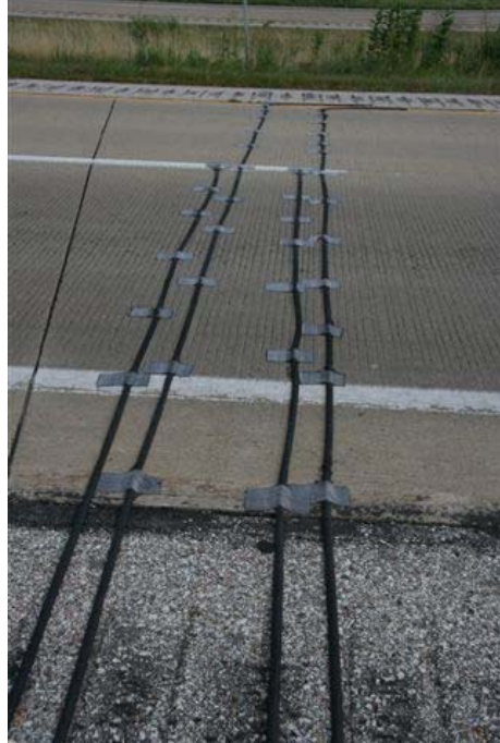
Figure 8. Position 1 setup (photo by Brad Grefe, CTRE)
