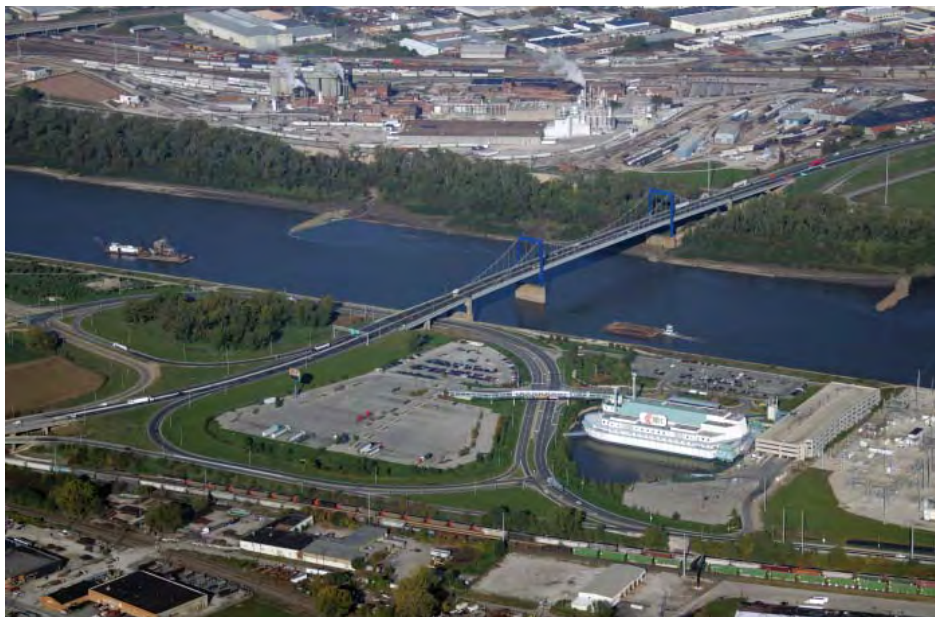
Aerial photo of the Paseo Bridge in Kansas City, Missouri
