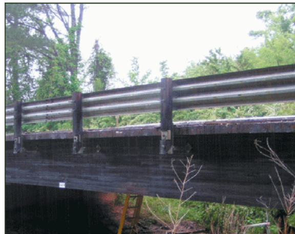
Figure 1. Transverse deck panels on glulam girders.
