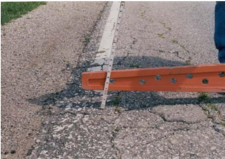
b. Close-up view of pavement damage resulting from edge loading.
