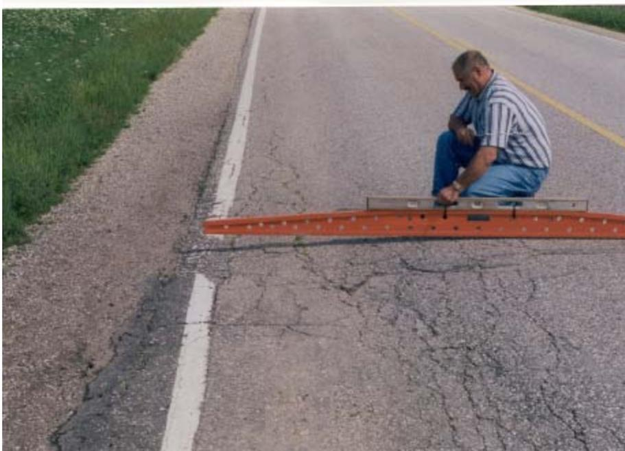
a. Overall pavement damage resulting from edge loading
